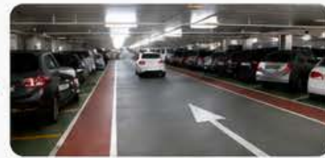
PU Carparking Flooring Applied
