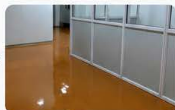
Screed Coat Applied Surface
