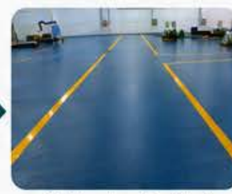
PU Flooring Applied (3mm to 4mm)
