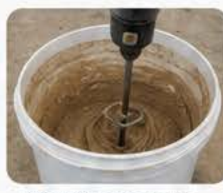
Mix All Components Thoroughly
