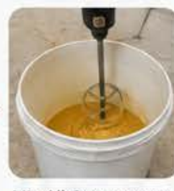
Mix All Components Thoroughly
